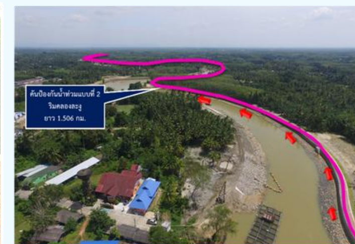
Retaining Wall (Flood Protection)
